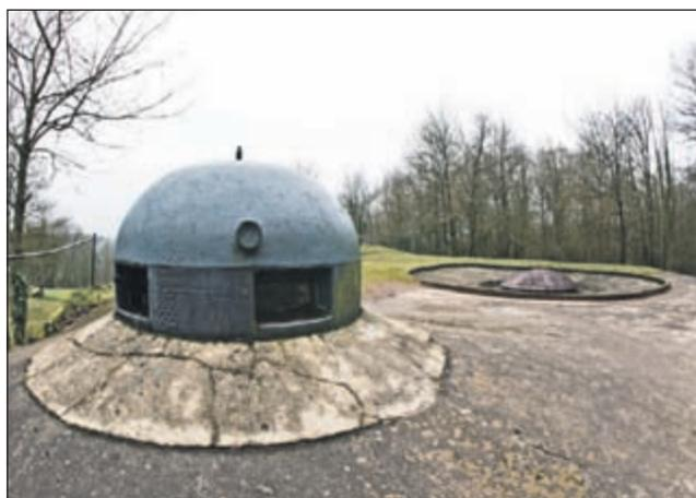
Observation cupola armed with two GFMs on the highest point on Block 9, behind right is a 135mm retractable gun.
